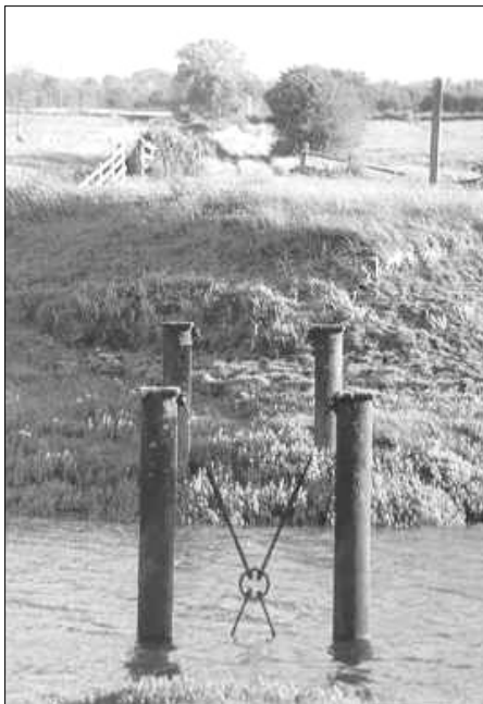
Piers of the bridge on the River Yeo, facing the site of Wick St Lawrence station
