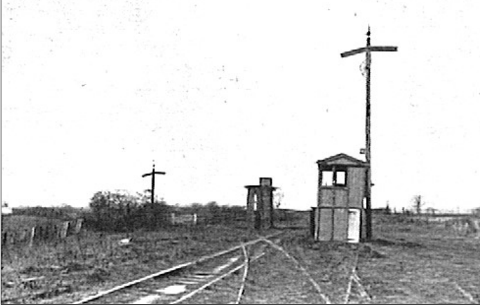
Kinnerley, Junction for the Criggion Branch, showing Ruined Signal Cabin, Signals and Water Tank.
