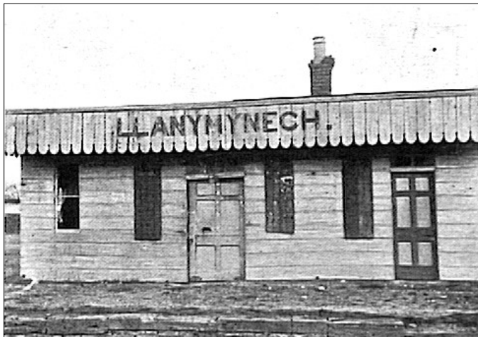
Station Office on Llanymynech Platform.
