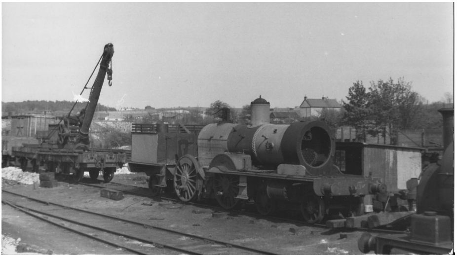
East Kent Railway, Shepherdswell, 5th May 1935 with Adams Radial Tank No. 5 under repair. Hand crane for lifting. Yes, No. 5 did work again! ( JHL Adams )
