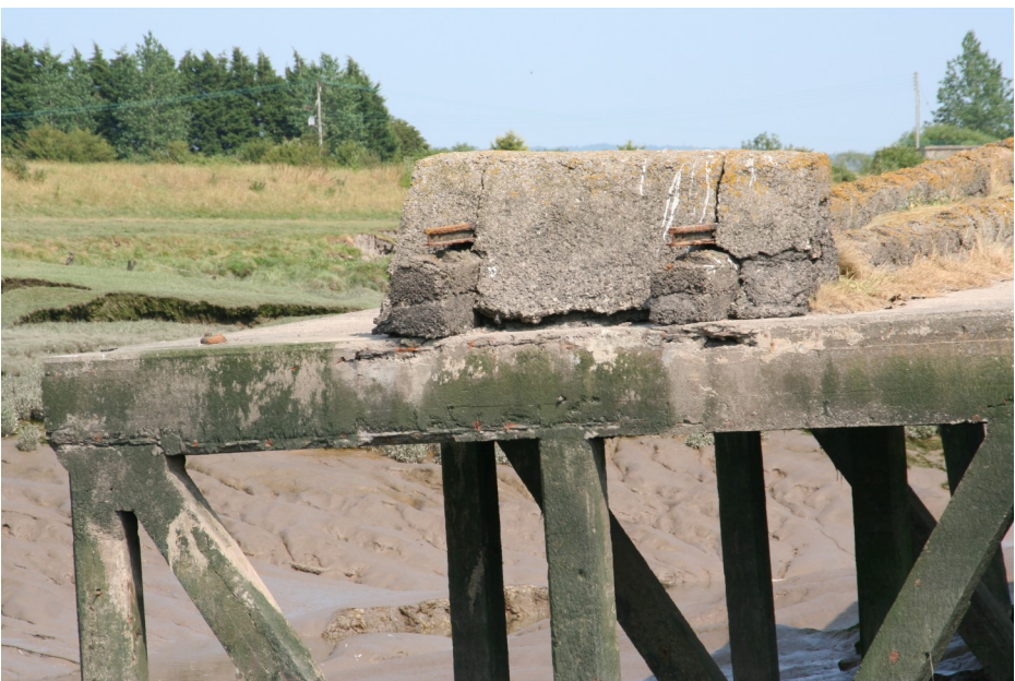
Two 2015 views of Wick St Lawrence Wharf on the WC&PR prior to raising the flood defences. The raised track bed due to subsidence is clearly visible. (Bob Edwardes)
