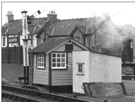
Not the frame in question, but the much cosier Ground Frame B at Callington, from one of Peter Barnfield's 1961 photos.
